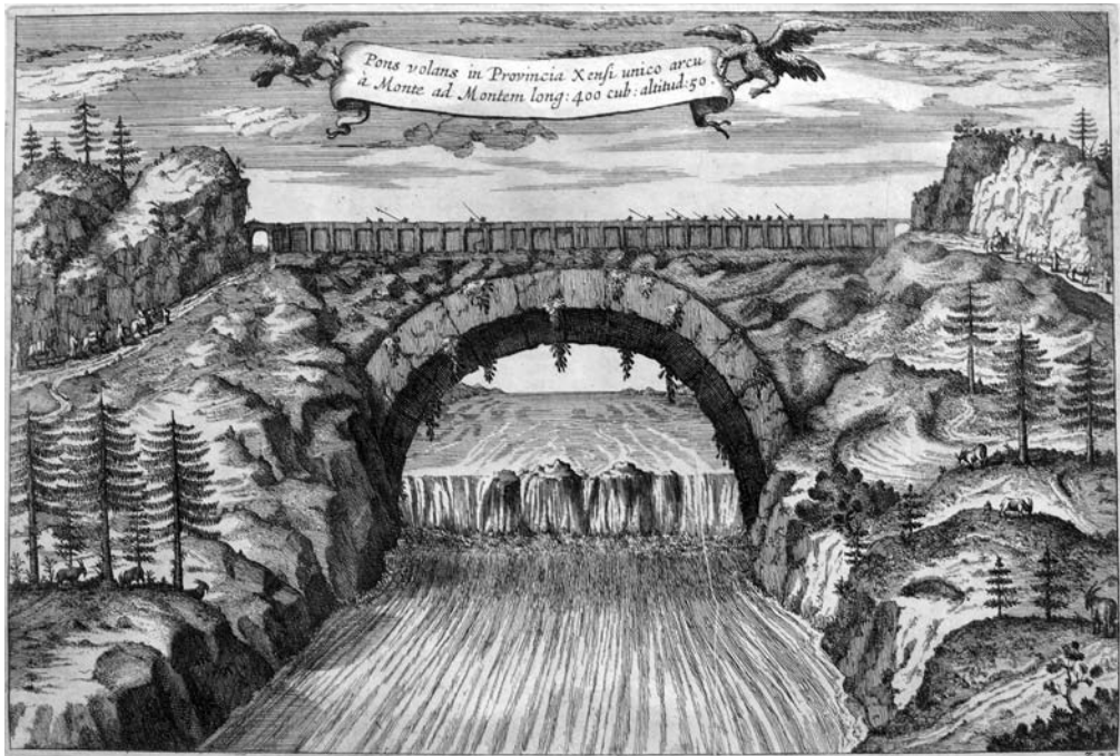
Cat. 17, facing p. 214, an example of Chinese bridge building
